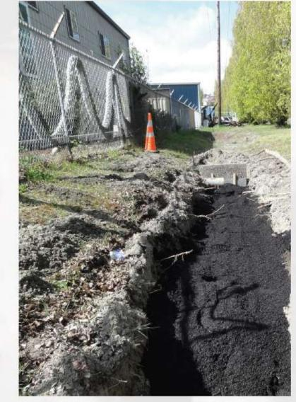
Figure 2: The Port of Port Townsend is using biochar to filter heavy metals in a below-grade swale. The galvanized fence in this photo is one of the boatyard's primary sources of zinc. (Image courtesy Francesco Tortorici)
